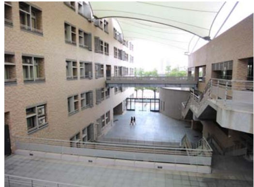
Management Building (inside)
